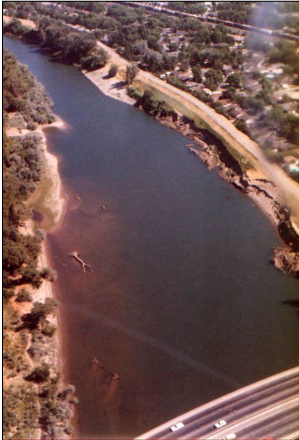
Figure 2-1. Left bank levee and riverbank erosion from 1986 flood event (134,000 cfs) upstream of Capital City Freeway
